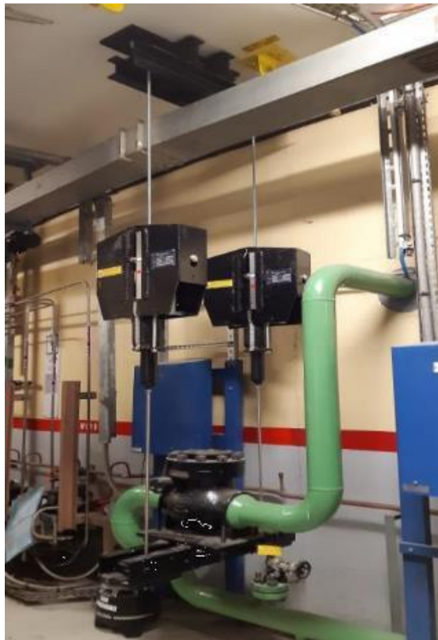
Renforcements tuyauteries ASG
